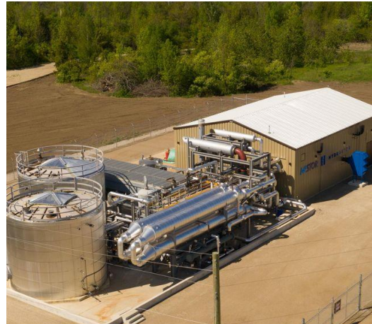
Illustration 4 Hydrostor's advanced compressed air energy storage pilot plant in Ontario, Canada (Source: Hydrostor)
