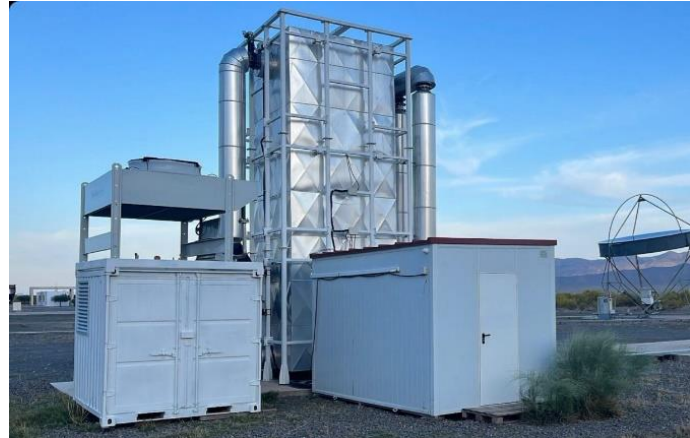
Illustration 5 Storenergy's pilot project is a 3 MWh TES system deployed in Spain. (Source: Storenergy)
